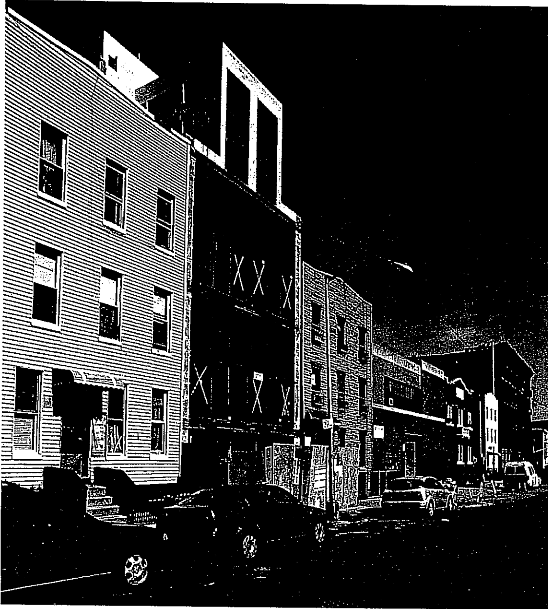
New housing construction in Williamsburg
